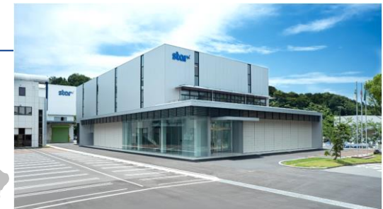
Completed in July 2020
